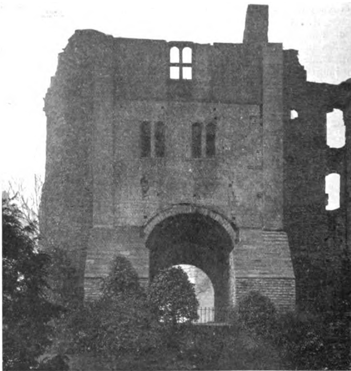
THE NORMAN GATEWAY OF NEWARK CASTLE. (Photograph by Mr. T. Richards, Newark.)
