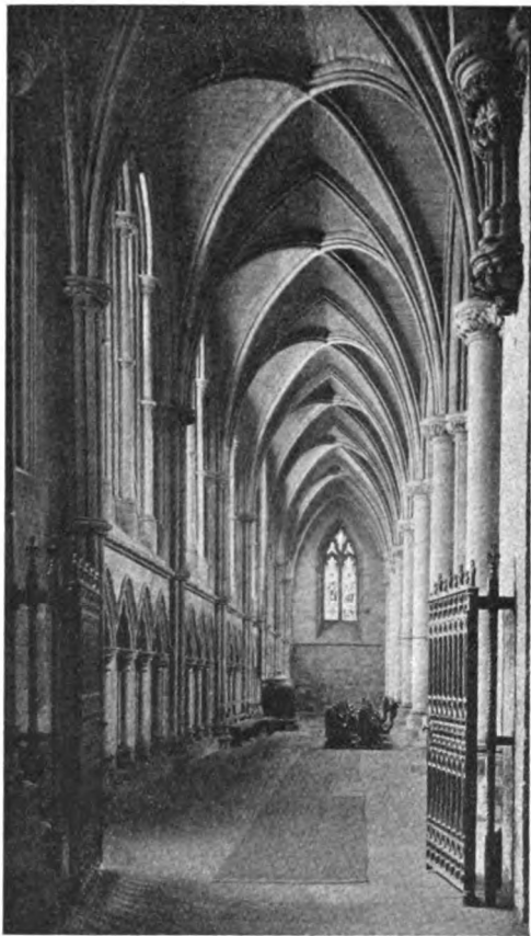
NORTH CHOIR AISLE, LOOKING EAST.
